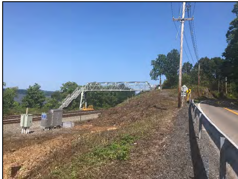
Path and MNR Pedestrian Overpass
