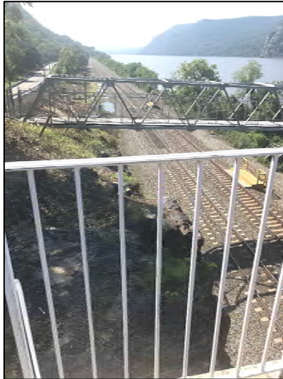
Ledge (rock cut) adjacent to MNR pedestrian overpass and observation platform
