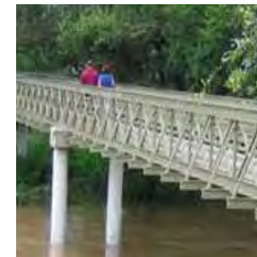
Fiberglass trail over a wetland
