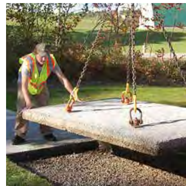
Installation of Storm-crete™ permeable unit pavers
