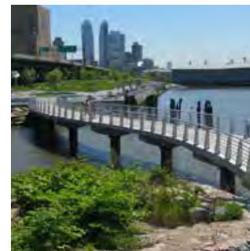
Concrete structure on piles
